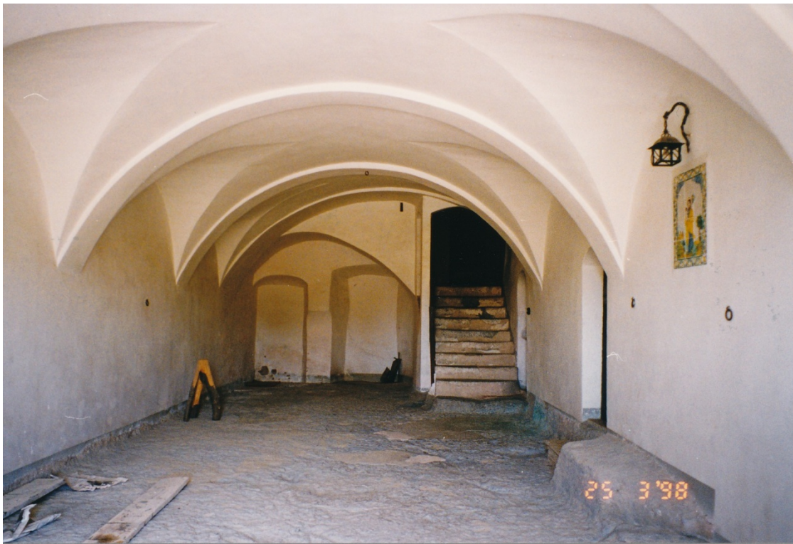
Cerda Downstairs. Under reconstruction— floor stripped to bedrock
